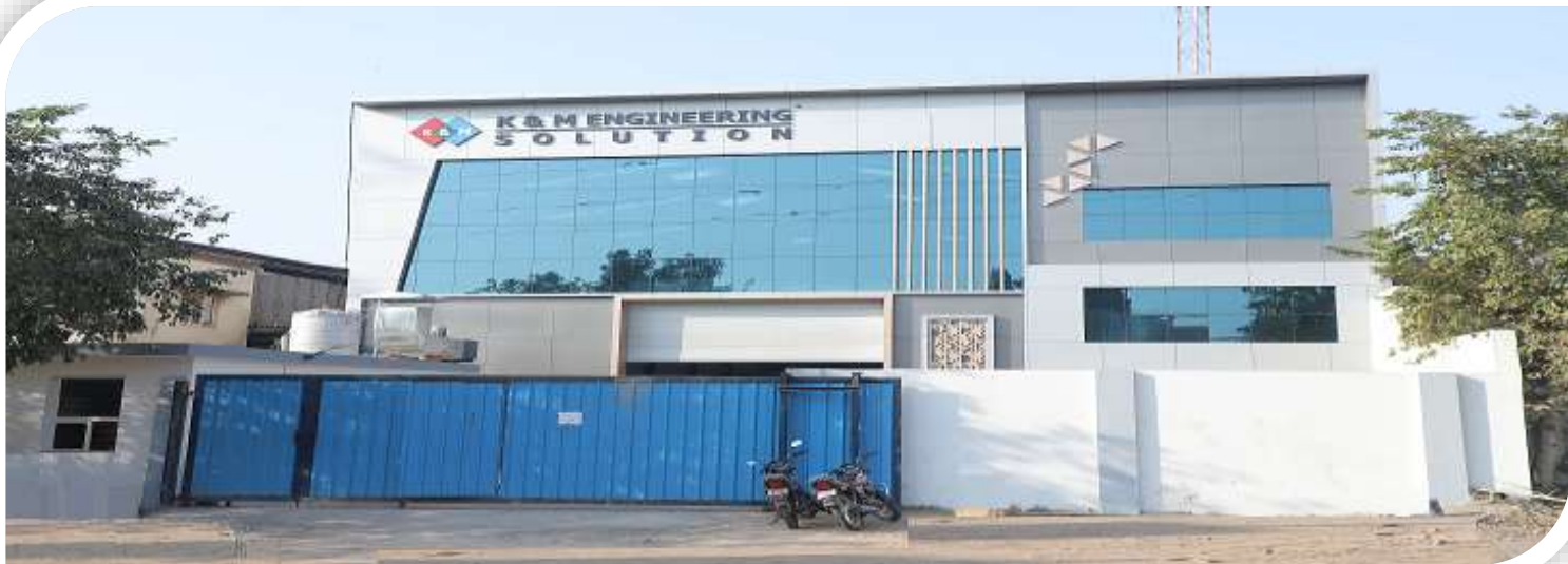
Unit -2 GIDC Vatva
