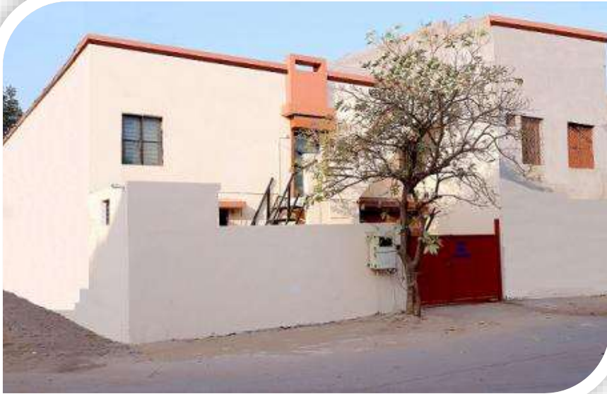
Unit -1 GIDC Vatva
